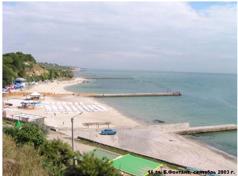
Fig. 4 View of the segment of the landslide protection from the second stage (1970s)
